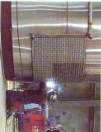
A.S.M.E. code thimble will be welded to a silo tank.
